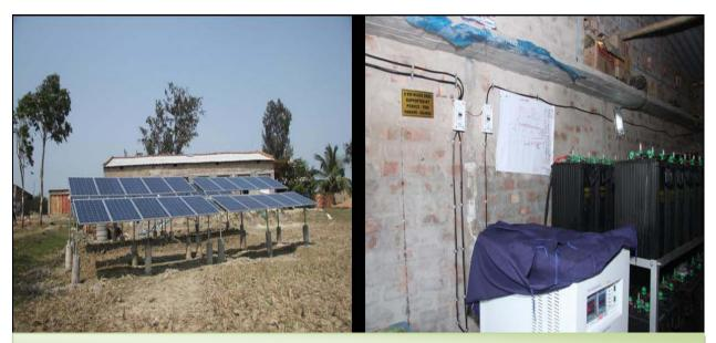
8kW plant and inverter & battery bank at Netaji Bazar
